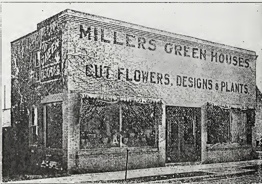
PLANT "A" WITH KILGORE AVENUE STORE.
